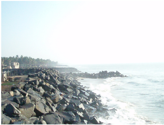
(a) Groynes at Kotakuppam.
